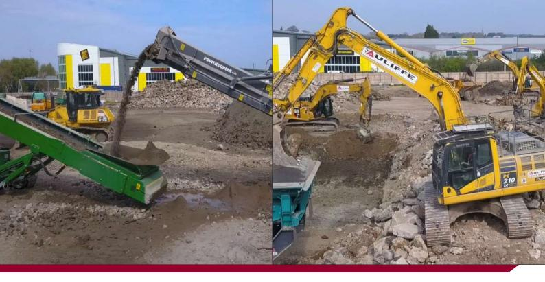
Before we started remediation, our team also demolished existing buildings onsite, stripping out asbestos fibres and removing all below-ground foundations and potential obstructions to future development.
